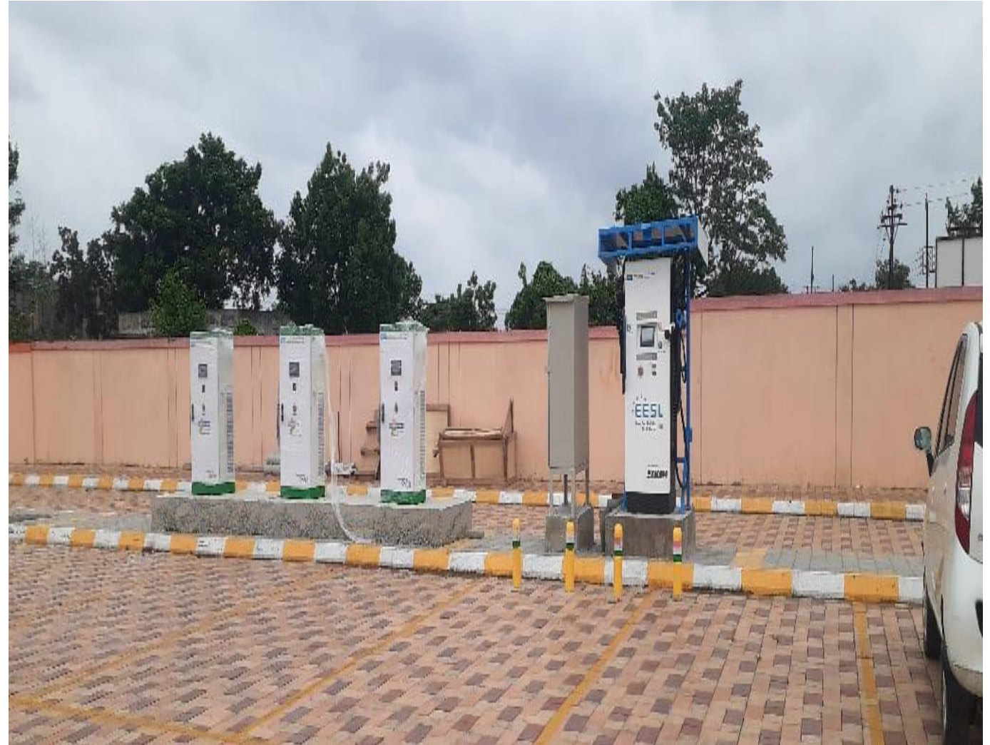
EESL charging stations at Khapri Metro Station
