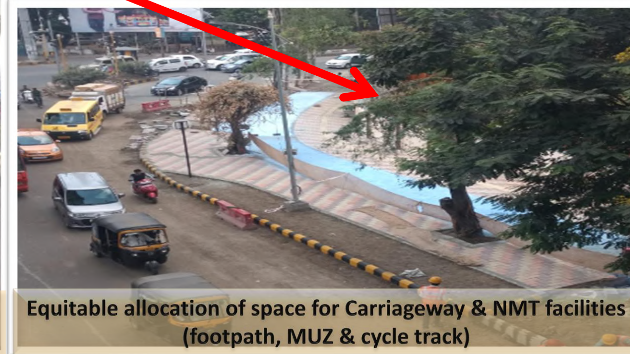
Equitable allocation of space for Carriageway & NMT facilities (footpath & cycle track)
