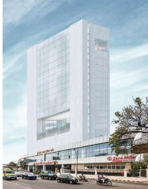
It is the first station of its kind in the country which has been designed as a 20-storey building with trains passing through its 4<sup>th</sup> floor. The building has two basement levels for parking exclusively. The building above the 4<sup>th</sup> floor where the platforms are located will have commercial development on PPP basis. People will be able to access the work areas above by lifts directly from the platforms.
