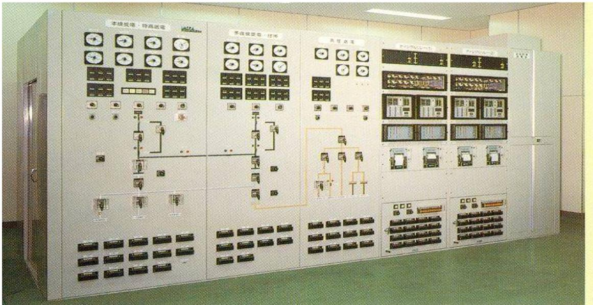
Fig. 9.2 : Typical Indoor Auxiliary Sub-station
