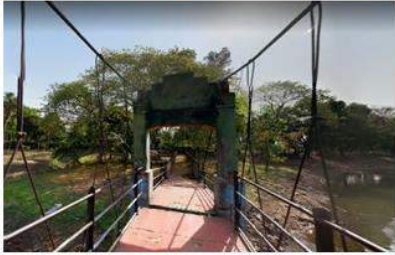
EXISTING SITE PICTURE
