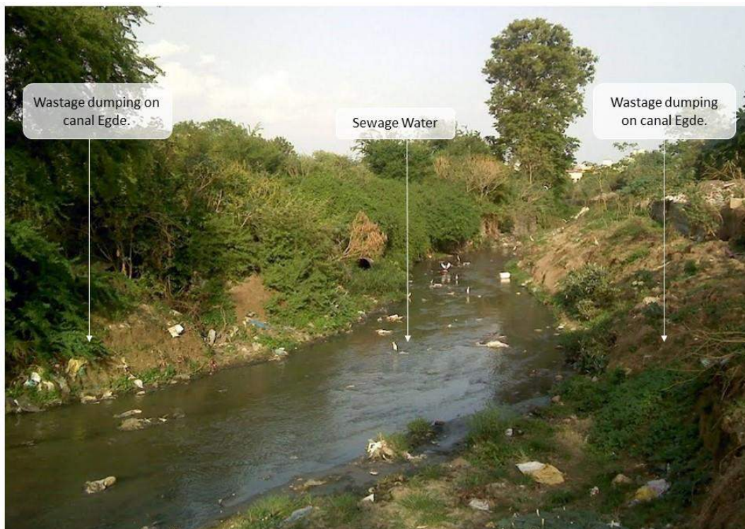
FIGURE B- 28 : EXISTING CONDITION OF THE NALLAH
