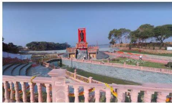
EXISTING SITE PICTURE
