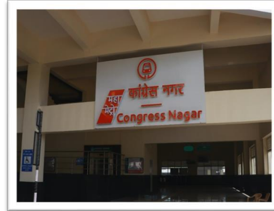
MAIN ENTRANCE OF CONGRESS NAGAR METRO STATION
