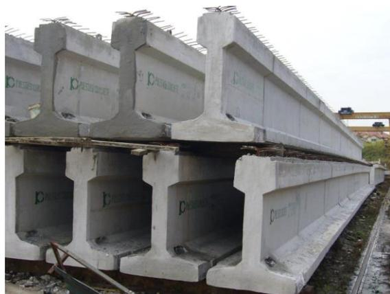
Box girder. Since unit length of I-Girder is for full span, their transportation is not possible for all locations. However, the unit weight of I-Girder is approximately in the range of 70 MT, which is almost half when compared to Double U-girder and hence can be launched with lower capacity road cranes. Deck Slab of I-Girder can easily be planned to accommodate curved alignment. I-Girders are most suitable for station locations, where Box and 'U' Girders are not continued.
