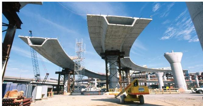
For Box girder segmental construction, normally span of 31m is kept by providing 9 segments of 3m length and two end segments of 2m length each. The other standard spans (c/c of pier) comprises of 25m, 28 m, 22m, 19m & 16m, which shall be made by removing/adding standard segments of 3.0m each from the center of the span.
