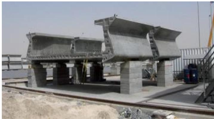
**d. Precast I-Girder Superstructure with Internal Pre-stressing**
