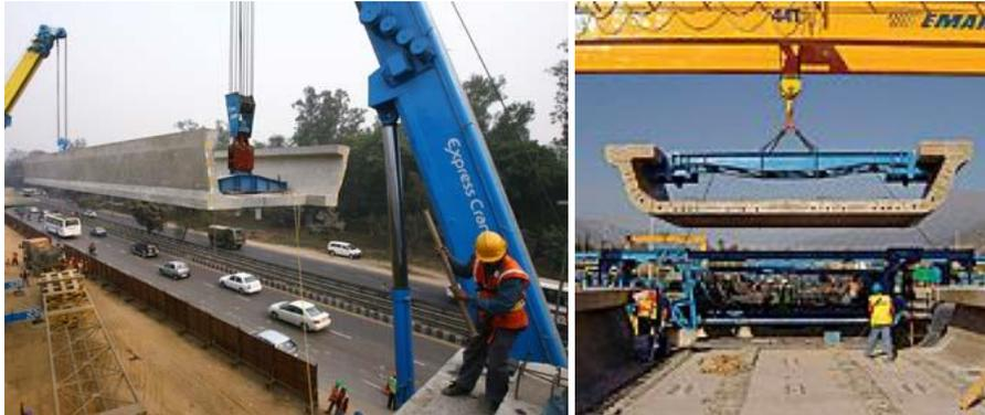
**c. Precast U-Channel Segmental Superstructure with Internal Pre-stressing**
