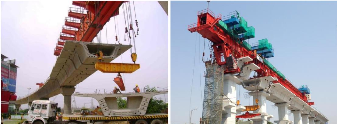
In such construction, the pre-stressing is placed outside the structural concrete (inside the box section) and protected with high density polyethylene tubes which are grouted with special wax or cement. The match cast joints at the interface of two segments are provided with shear keys as in traditional segmental construction.
